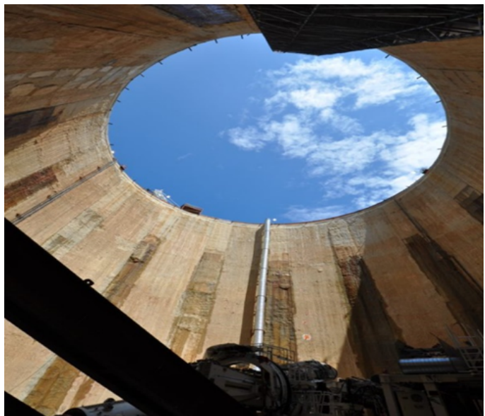
Clean Rivers Tunnel Construction Shaft
