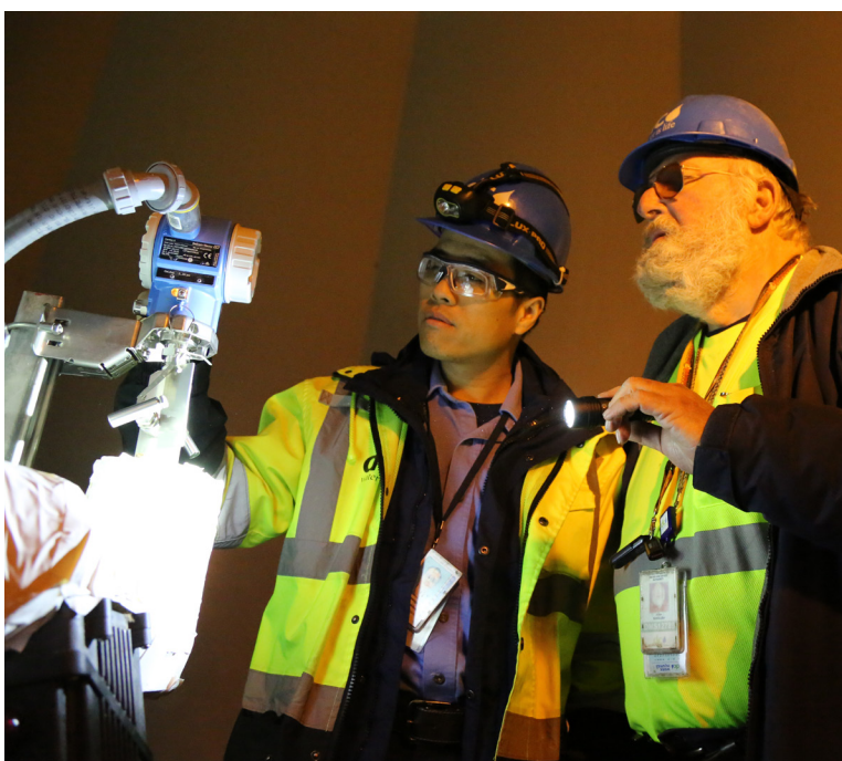
Anacostia Pumping Station inspection
