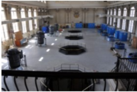
Main Pumping Station
