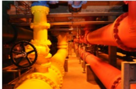
Anacostia Pump Distribution Systems
