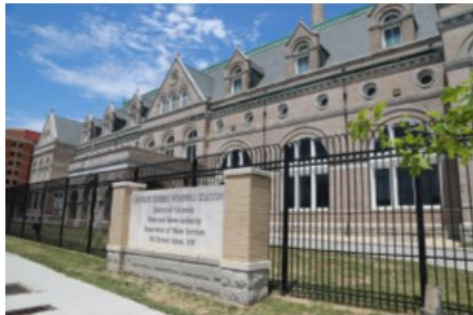
Bryant Street Pump Station
