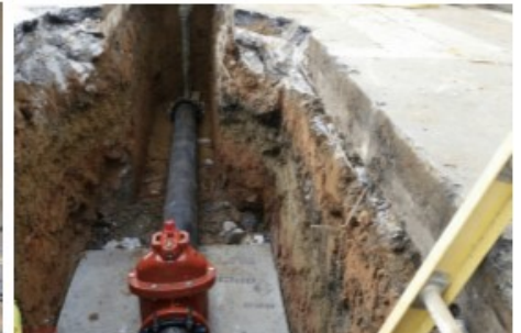
Small Diameter Replacement Program
