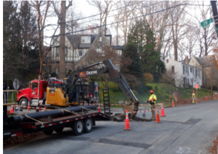
Small Diameter Water Main Repair
