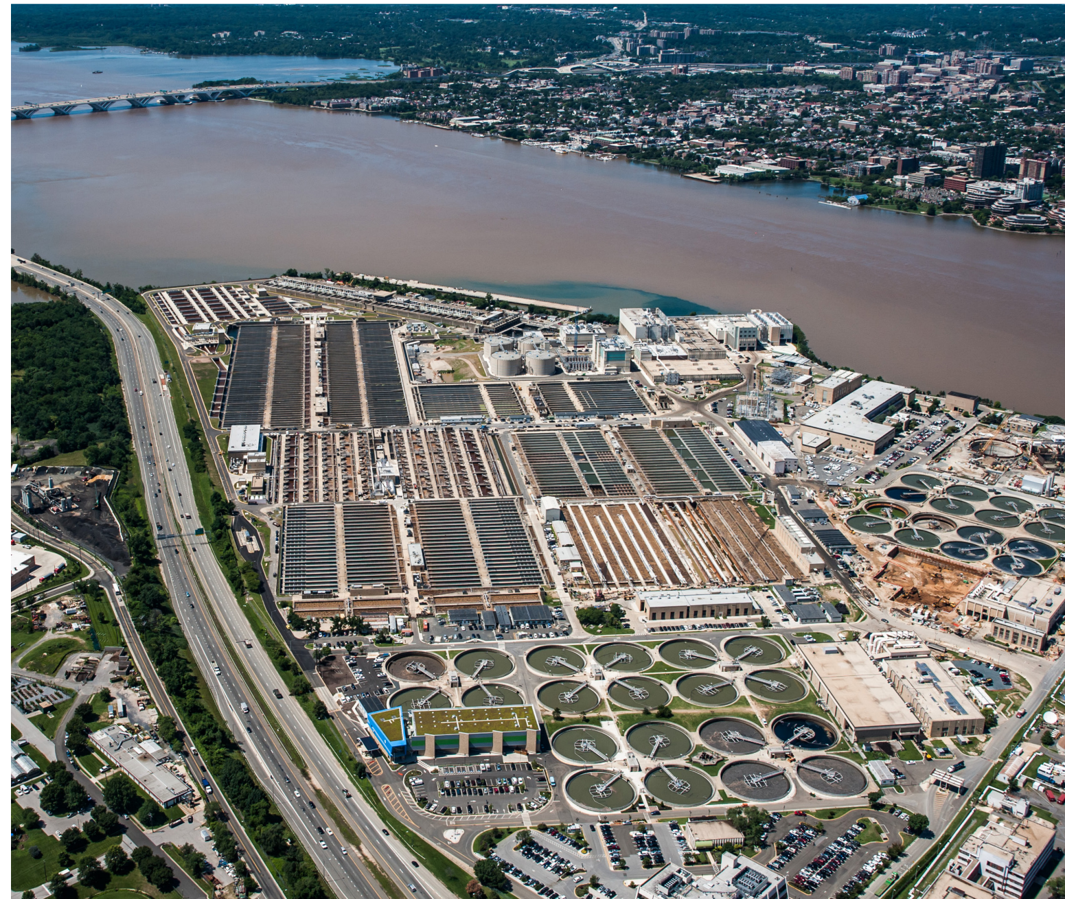
Blue Plains Advanced Wastewater Treatment Plant
