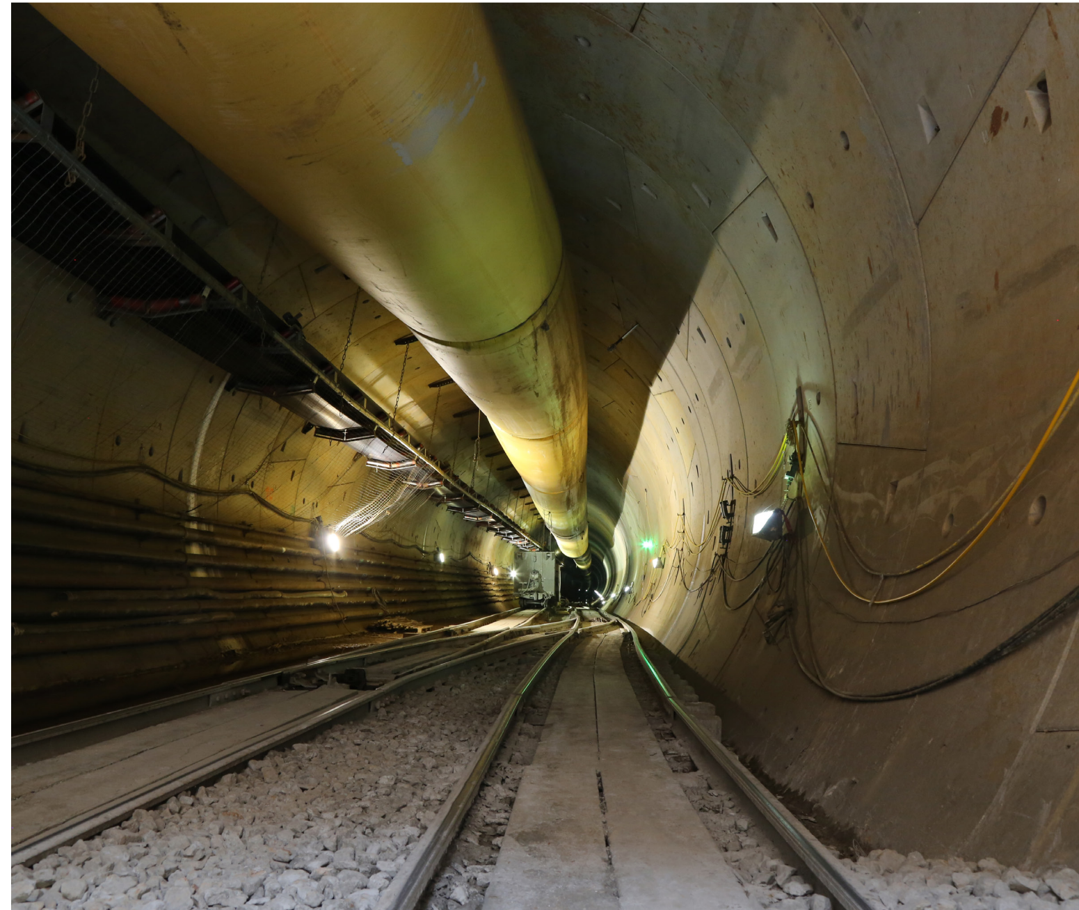
DC Water Clean Rivers Project – Anacostia River Tunnel River System
