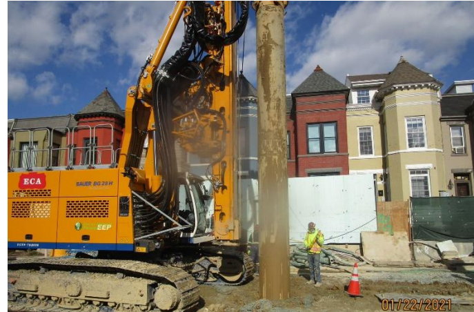
T Street - Soldier Pile Installation DCCR
