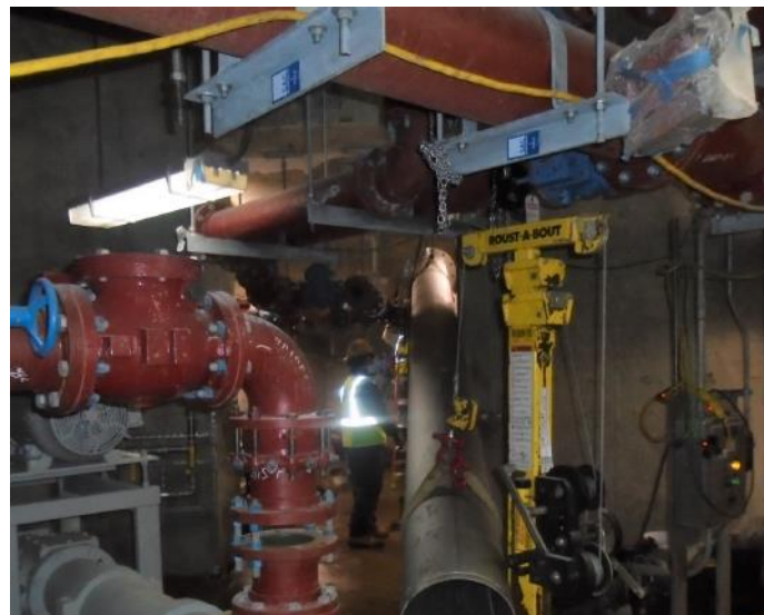
Blue Plains Gravity Thickener Upgrades
