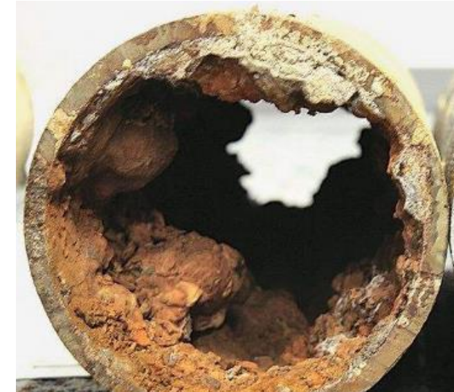
SDWM unlined Cast Iron pipe
