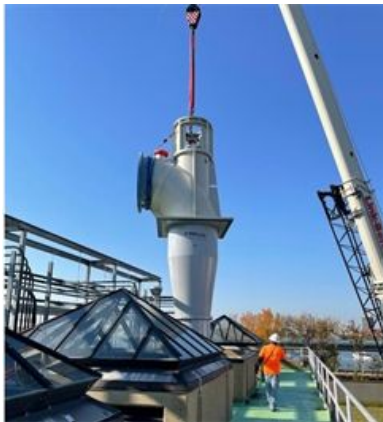
Filter Influent Pump Installation
