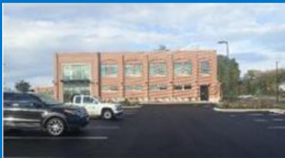
Sewer Services Facility
