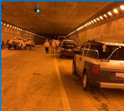
Third Street Tunnel Water Main Repair
