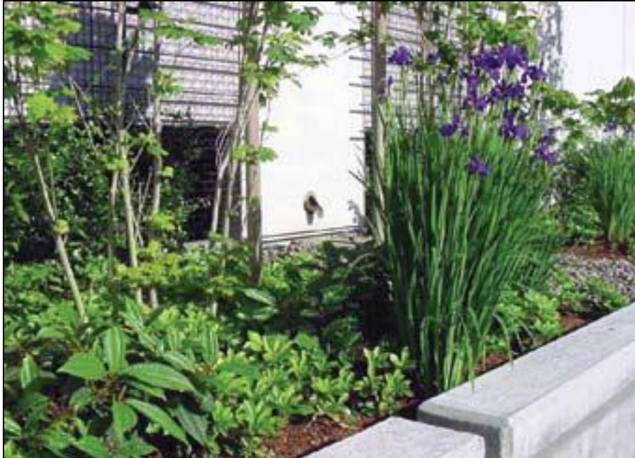
Figure 2-5. Typical bioretention planter box adjacent to a building.
