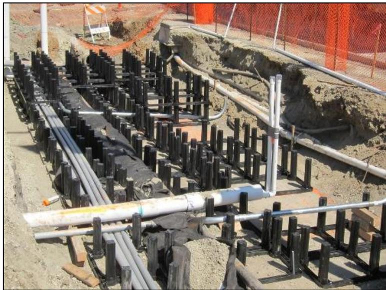
**Figure 4-8. Utilities placed within Silva Cells.**
