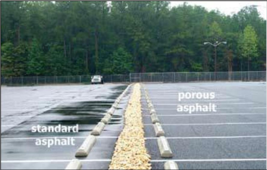
Figure 3-12. Porous and conventional asphalt.
