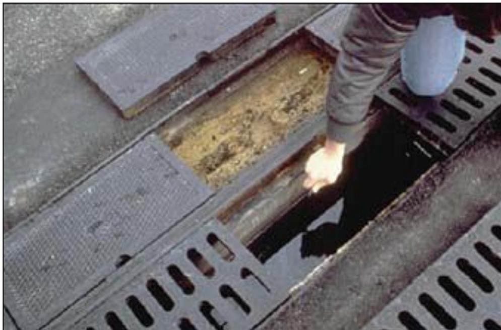
**Figure 9-8. Access for maintenance of perimeter filter system.**
