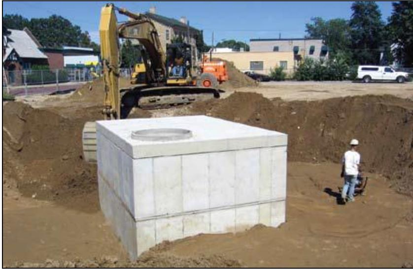
**Figure 7-4. Multiple underground cisterns in series.
