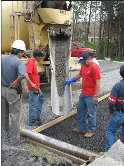
**Figure 3-5. Placement of pervious concrete.**
