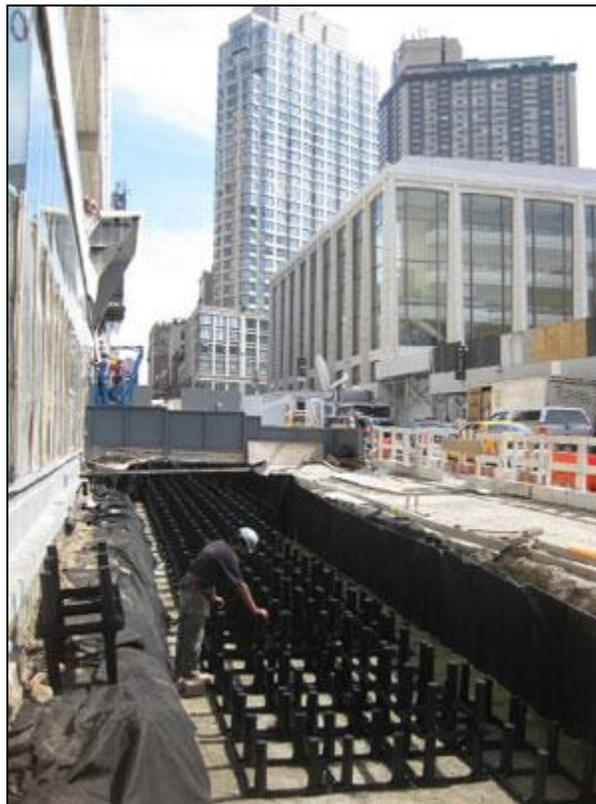
**Figure 4-5. Installation of Silva Cells at Lincoln Center
