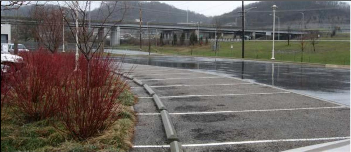
**Figure 3-9. Pervious concrete in parking lot stalls.**
