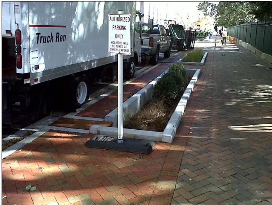
**Figure 2-6. Bioretention planters adjacent to a roadway in Richmond, VA.
