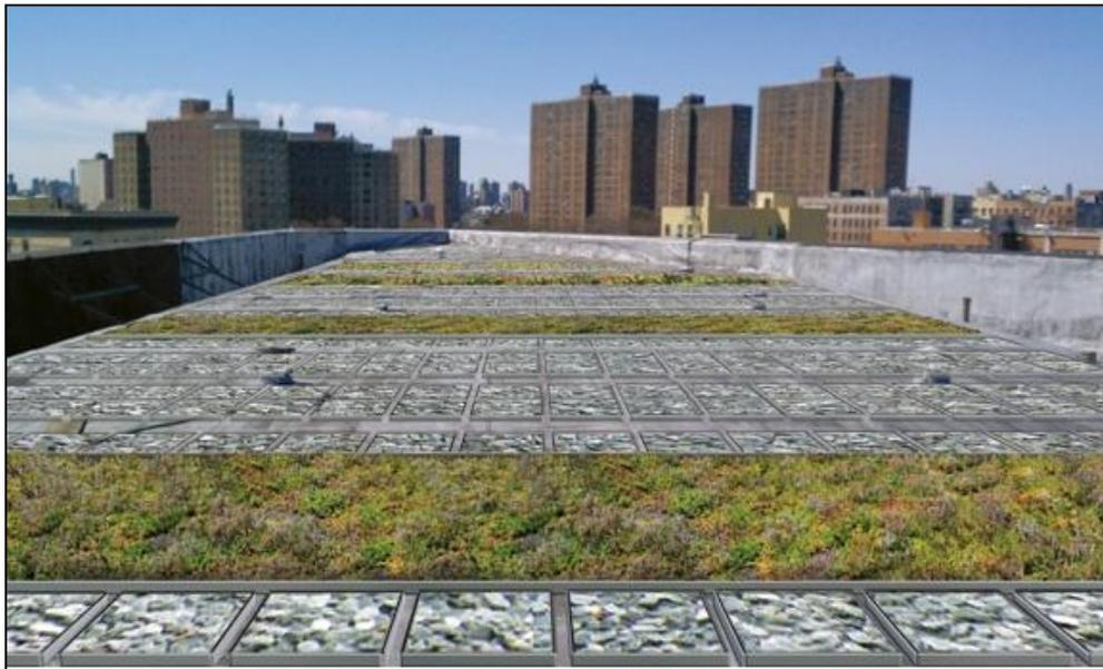
**Figure 8-6. Blue roof installed in combination with green roof, New York, NY.
