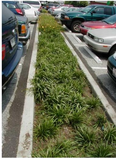
**Figure 3-4. Navy Yard Bioretention Strip**
