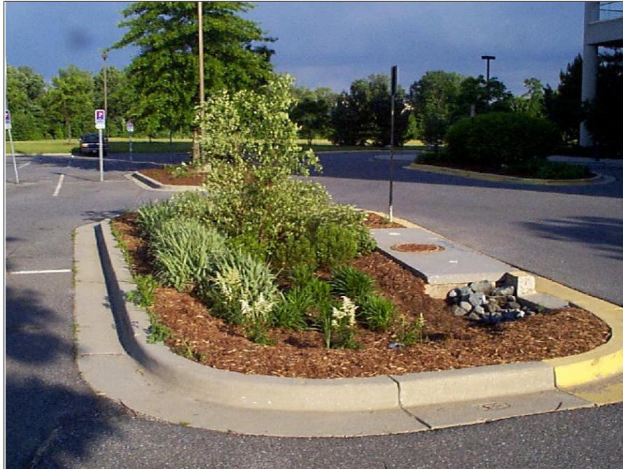
**Figure 2-8. Bioretention in a parking lot island.**
