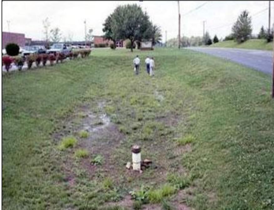
**Figure 9-9. Sand filter application with vegetation.**
