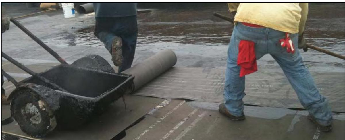
**Figure 8-7. Installation of a waterproof membrane during blue roof construction.
