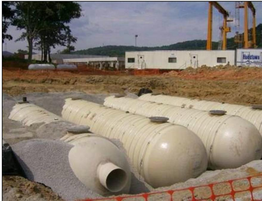
**Figure 7-3. Multiple underground cisterns in series.**
