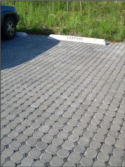
**Figure 3-14. Pervious pavers in parking area.
