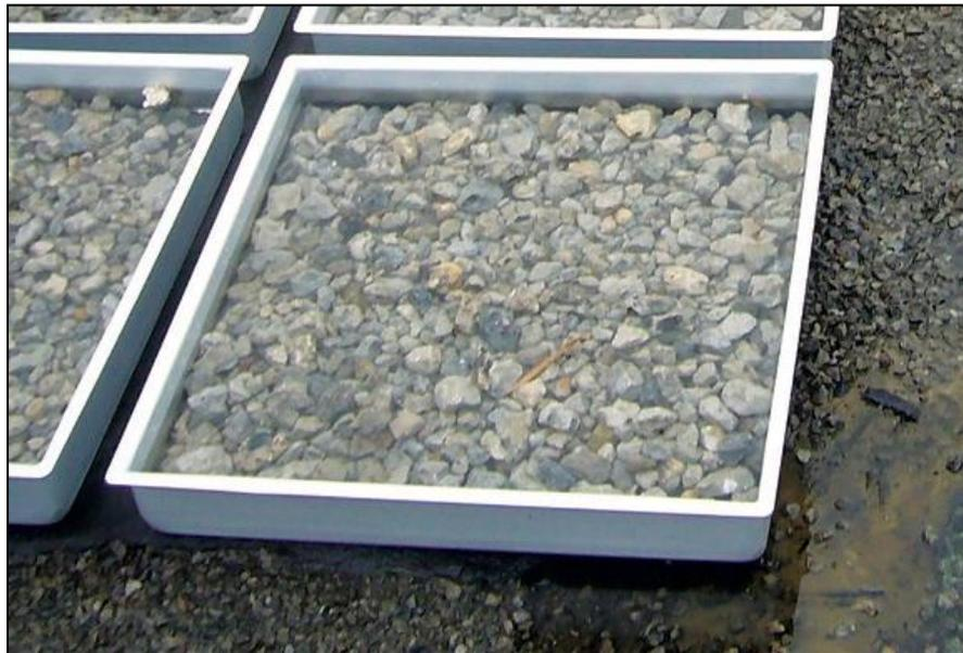
**Figure 8-5. Typical blue roof modular tray with gravel ballast.**
