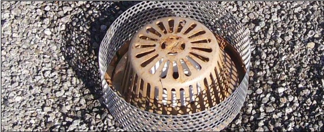
**Figure 8-3. Strainers or screens help prevent debris from clogging roof drains.**
