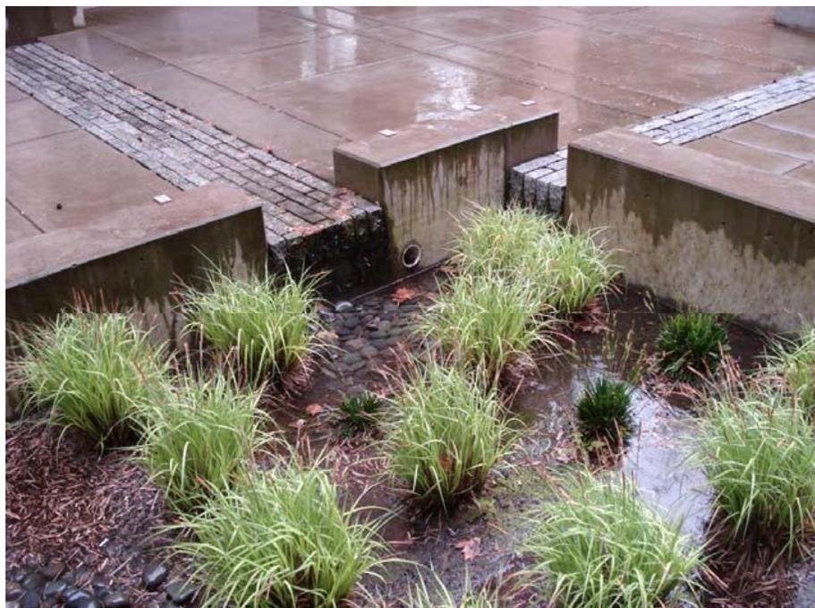
**Figure 2-7. Bioretention planter in an urban courtyard.
