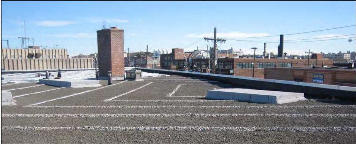
**Figure 8-2. Check dams installed to control flow on sloped portion of roof, Brooklyn, NY.
