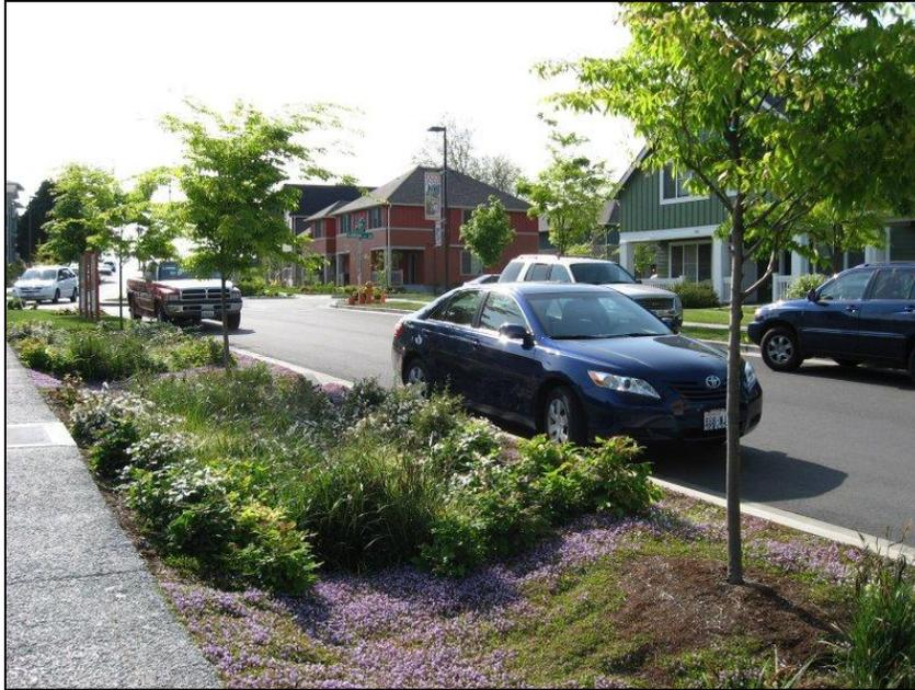
**Figure 5-2. New residential street uses a vegetated swale to capture runoff.
