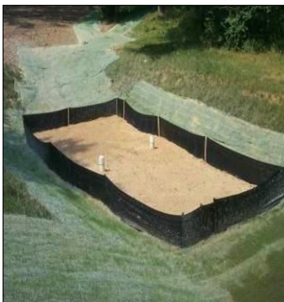
**Figure 9-2. Surface sand filter during construction
