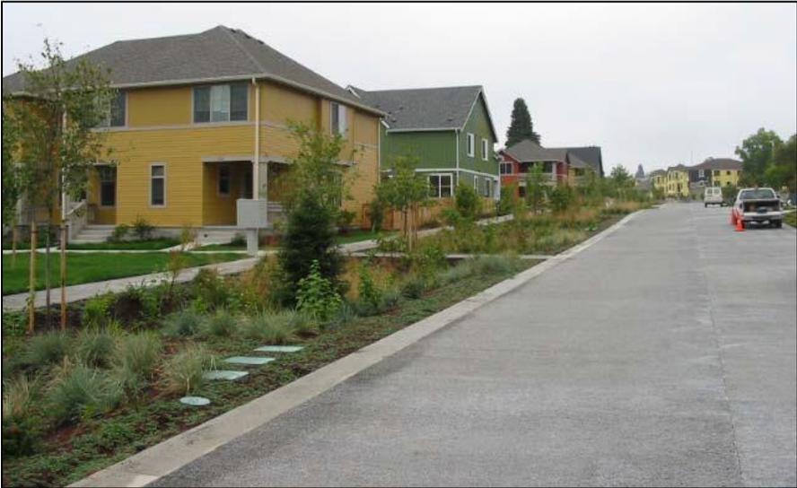
Figure 3-13. Pervious concrete residential street.
