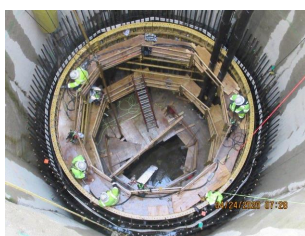
View down the drop shaft
