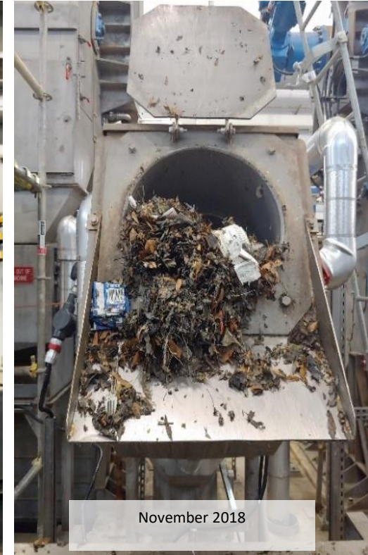
Trash and debris removed from CSO captured by tunnel at ECF Fine Screens
