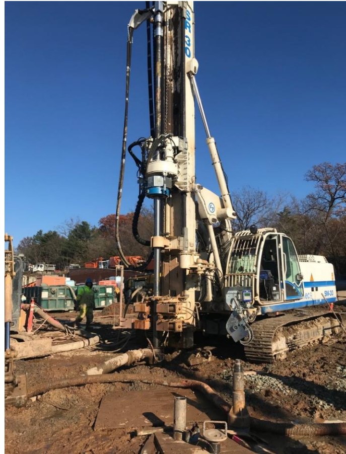
Jet Grout Rig
