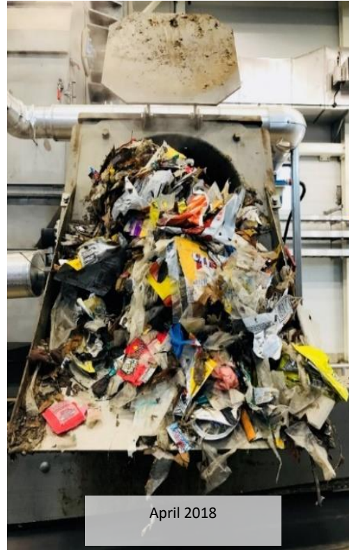
Trash and debris removed from CSO captured by tunnel at ECF Fine Screens
