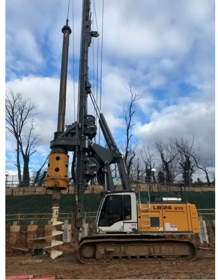
Caisson Drill Rig
