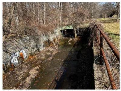
Photo 2: Former single-gate outfall was converted to a double-gate outfall in 1957 (Traceries, 2022).
